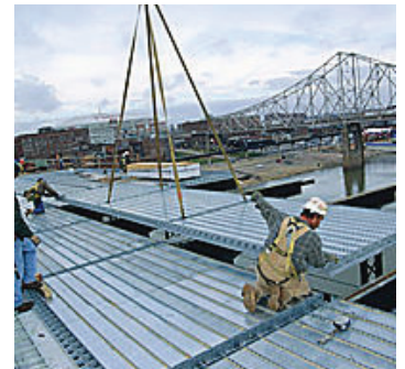
Exodermic™ Install, Eads Bridge
