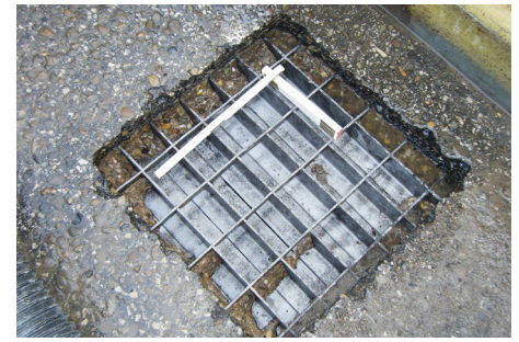
Inspection area of the 10th Street Bridge
