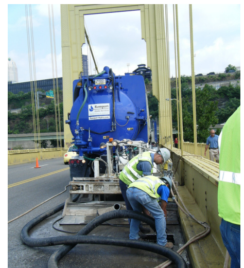
Inspection of the 10th Street Bridge Deck
