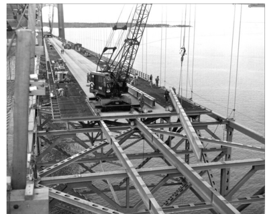
Construction on the Mackinac Bridge
