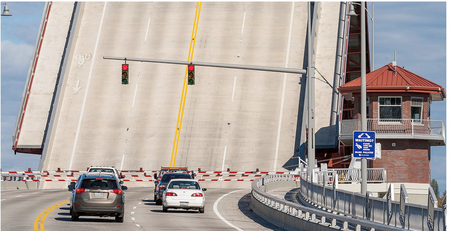
South Park Bascule Bridge Photos Courtesy of HNTB.
