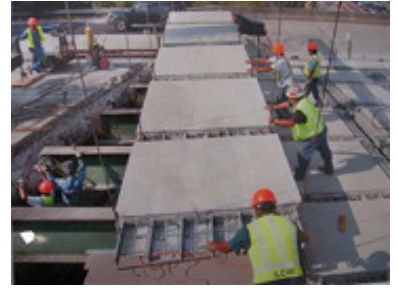
I-75 - Grid Deck Construction (Photo Courtesy of L.C. Whitford)
