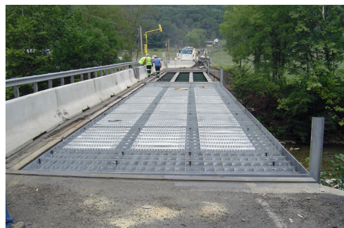
Exodermic Deck being Installed
