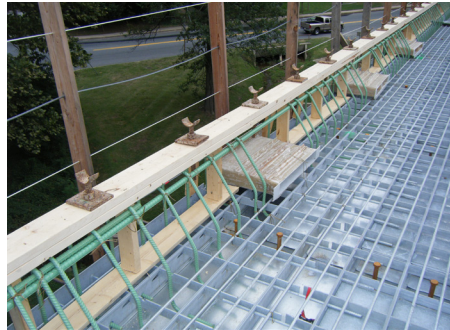
Barrier Reinforcement in Place
