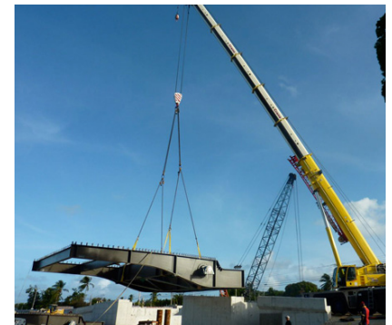
Lifting Section of Bridge (Photo Courtesy of Crane & Equipment Ltd.)
