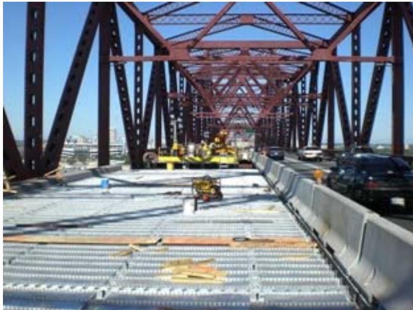
Figure 5. Bare Exodermic™ panels placed on Mathews Bridge.
