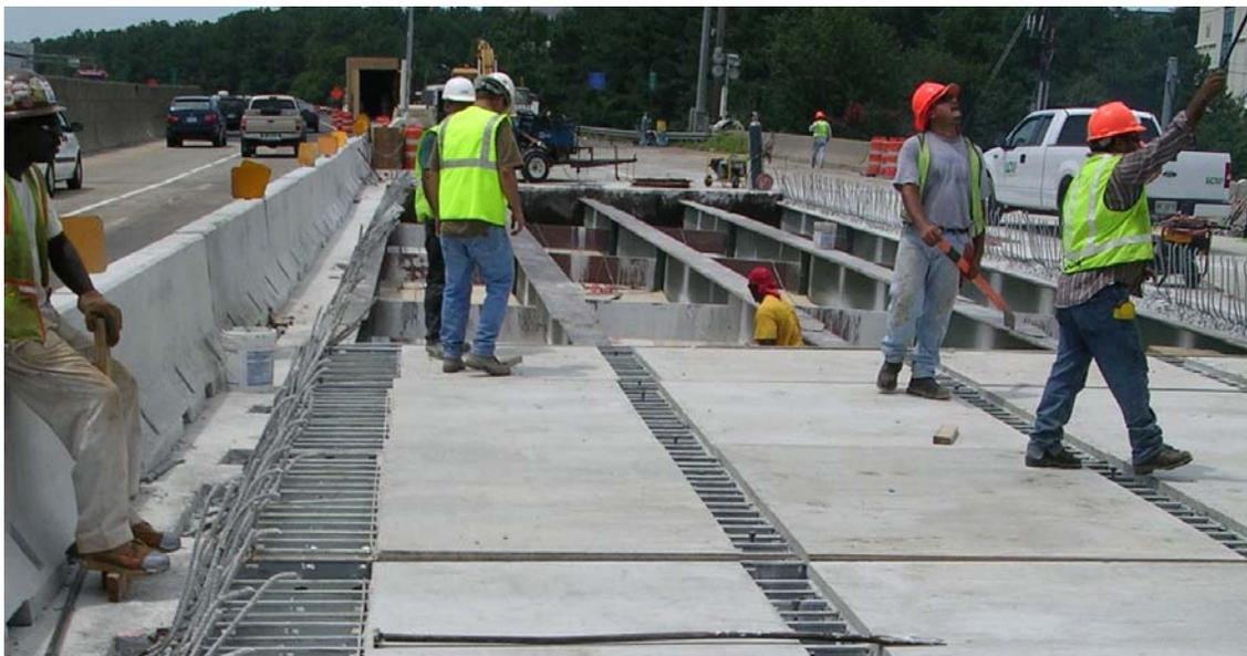
Figure 4. Precast panel installation on I-285 near Atlanta, GA.
