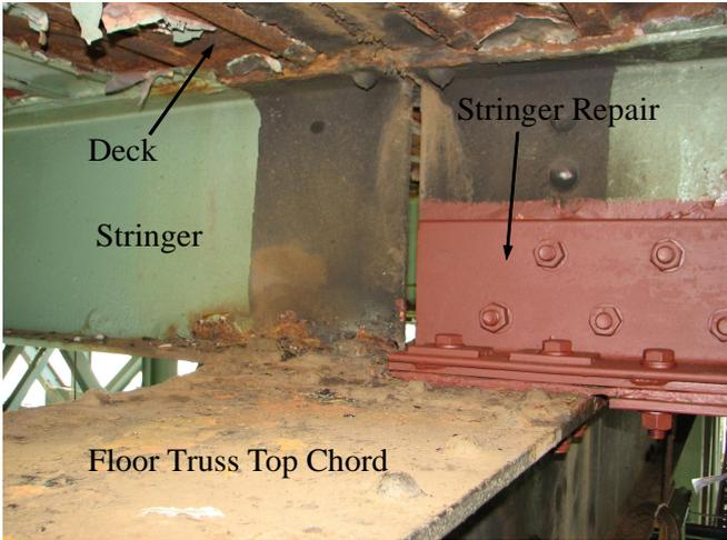
Figure 3: Deterioration in Deck, Stringers and Floor Trusses
