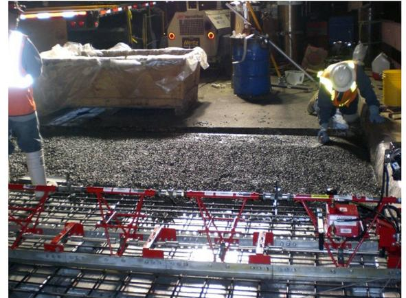
*Mathews Bridge in Jacksonville, FL where lightweight concrete was used in conjunction with an Exodermic™ deck to further reduce weight. The deck weighs less than 50 pounds per square foot while maintaining 2 inches of concrete cover over the rebar.*
