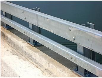
Combination concrete parapet and metal railing.
